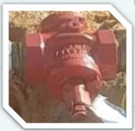
turn off the gas, these valves need to be in the closed position. With the use of 12 to 15" adjustable pipe or crescent type wrench or other suitable tools for specific valves, operate these valves a quarter turn in either direction. These valves will be closed when the handle or part you put the wrench on (the tang) is crosswise to the pipe.
