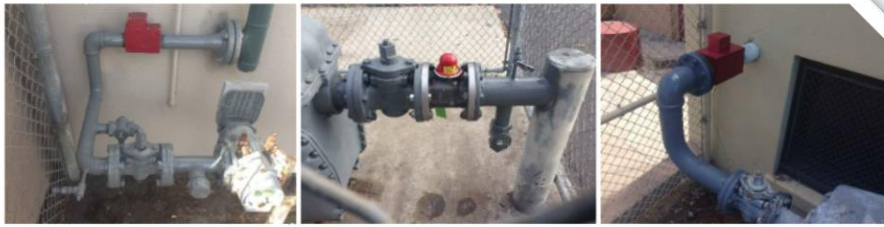
Completed work at Piedmont USD
